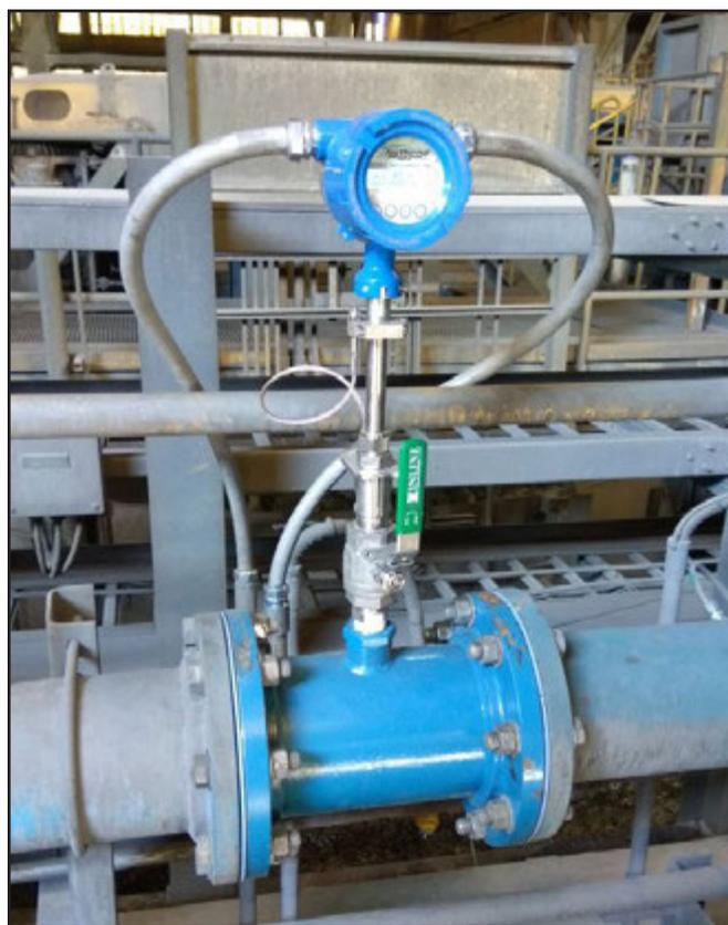
*Fox Thermal Model FT4A thermal mass flow meter and temperature transmitter.*
